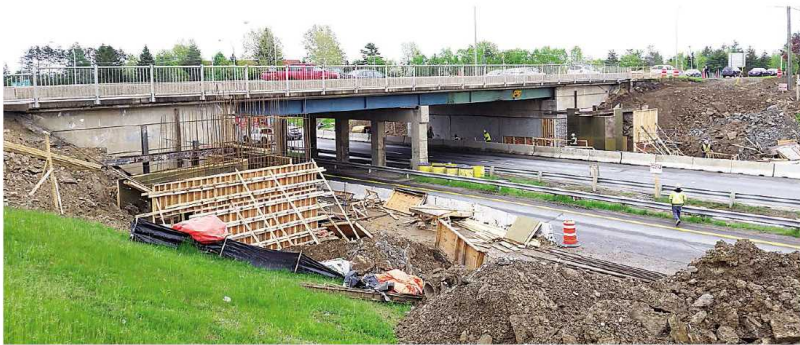
On Wednesday, the Regent Street overpass will close until the end of August to allow the provincial government to raise and widen it. The intersection of Regent and Prospect streets will also be reduced to one lane for three months while it's raised and widened by the province. PHOTO: STEPHEN LLEWELLYN/THE DAILY GLEANER
