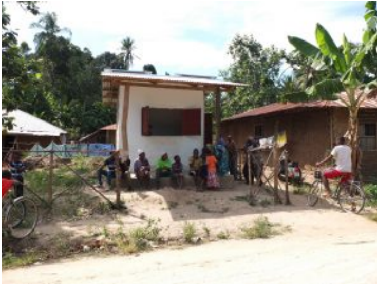
An outside view of one of the Jaza charging stations. Image: Submitted
